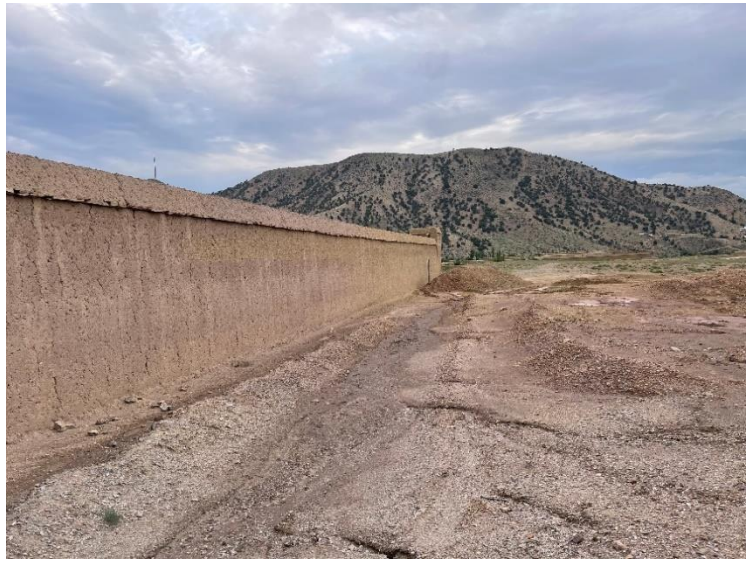
Figure 2-9 Length to height ratio of Pakhsa walls
