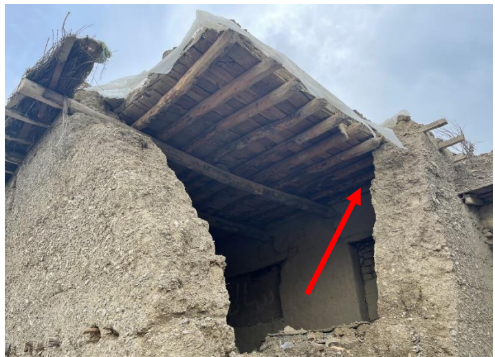
Figure 2-12 Example of Pakhsa wall construction
