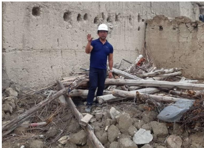
Figure 4-2. A high volume of salvageable timber at an assessed site.
