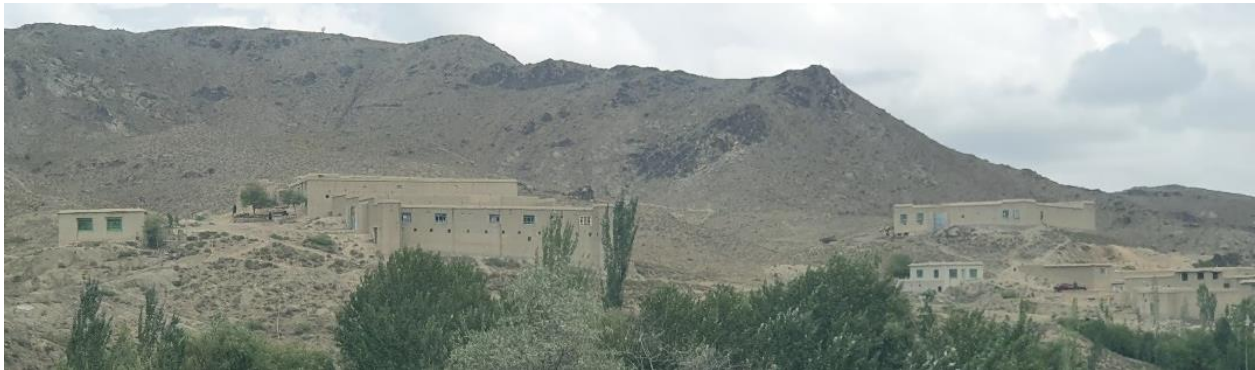
Figure 2-4. Views across remote valleys in the region with few signs of introduced modern building materials.
